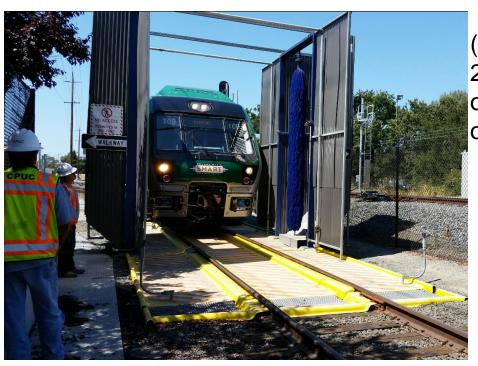
(1) Wash rack clearance issue. GO 26-D section 9.2. requires clearance of 30 inches from widest car operated.
