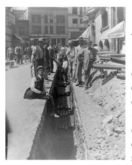
(Ca. 1897) – An Edison Electric crew is laying conduit for one of LA's earliest underground electric distribution systems.
