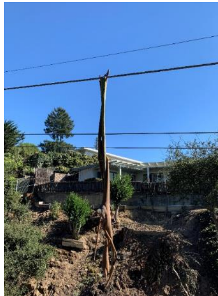
Figure 17: Image of Vegetation Hazard in Alameda County - Tree Limb Fell onto Conductor
