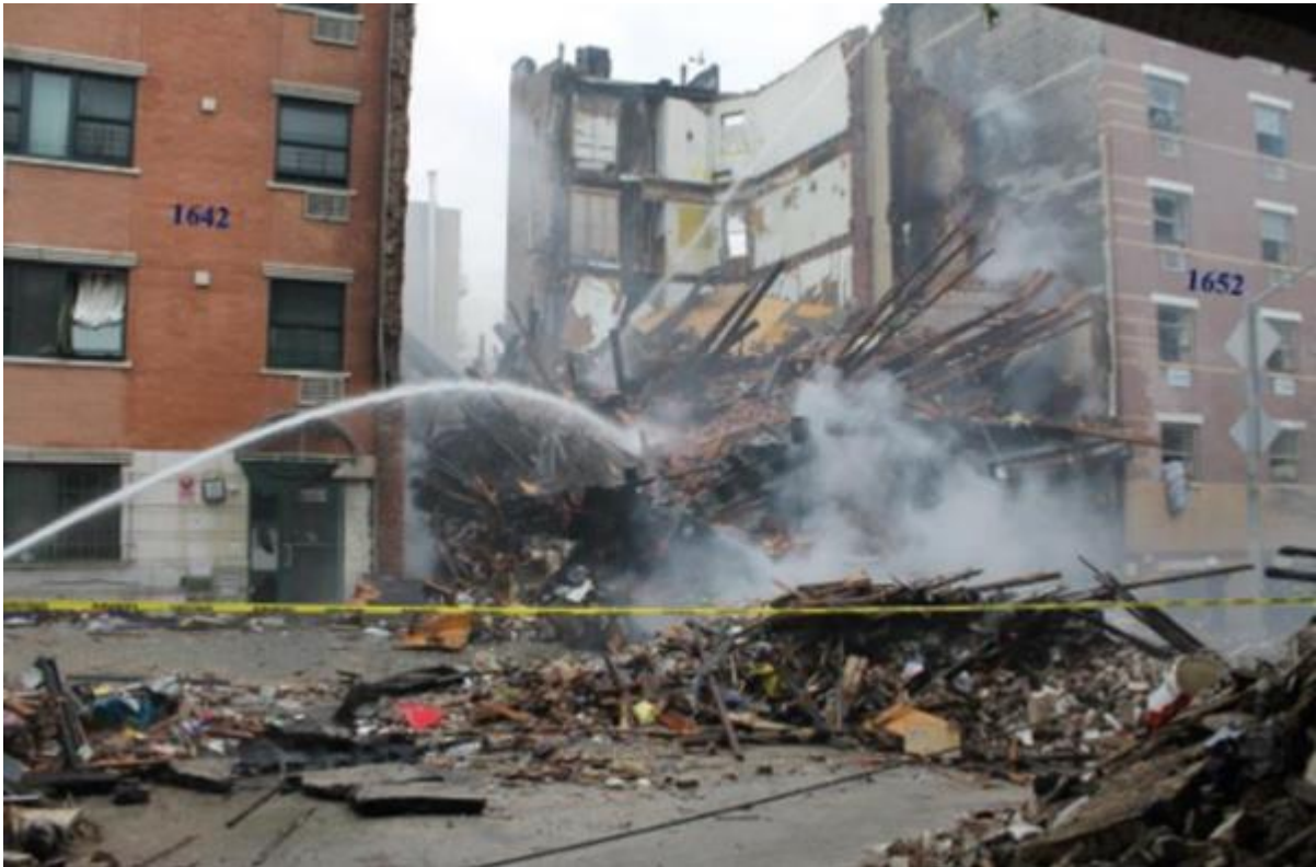
FIGURE 2-3 2014 EXPLOSION IN NEW YORK
