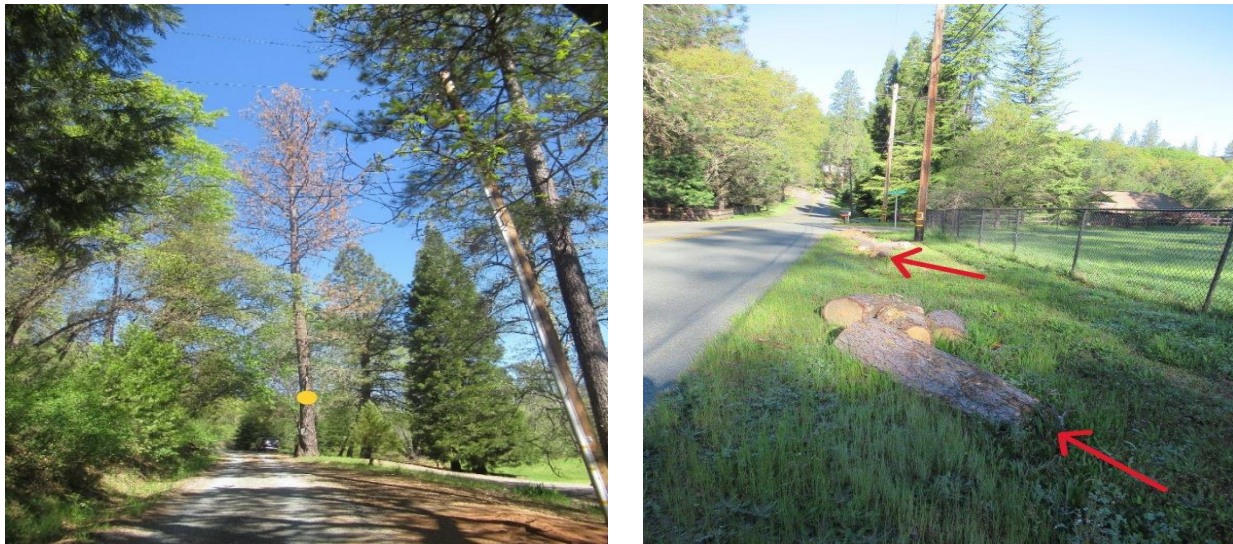
Figure 14: Left: Dead ponderosa pine not identified as a hazard tree in post storm investigation; Right: Wood management deviations from ANSI BMPs
