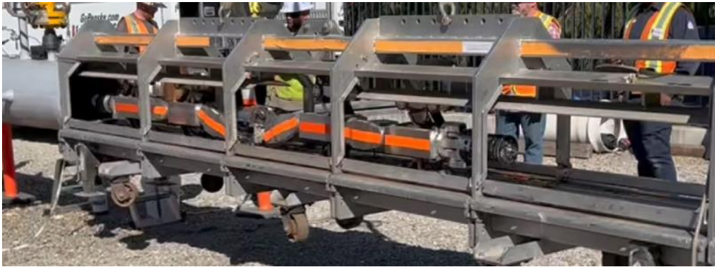
Figure 22: Loading of the robotic ILI tool via a carrier sled.
