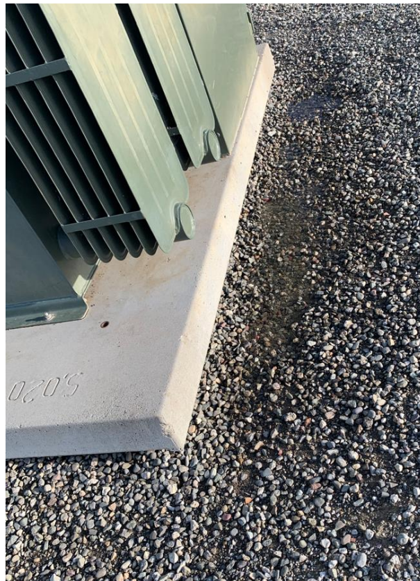
Figure 10. Base of padmount transformer at WTG F4.
