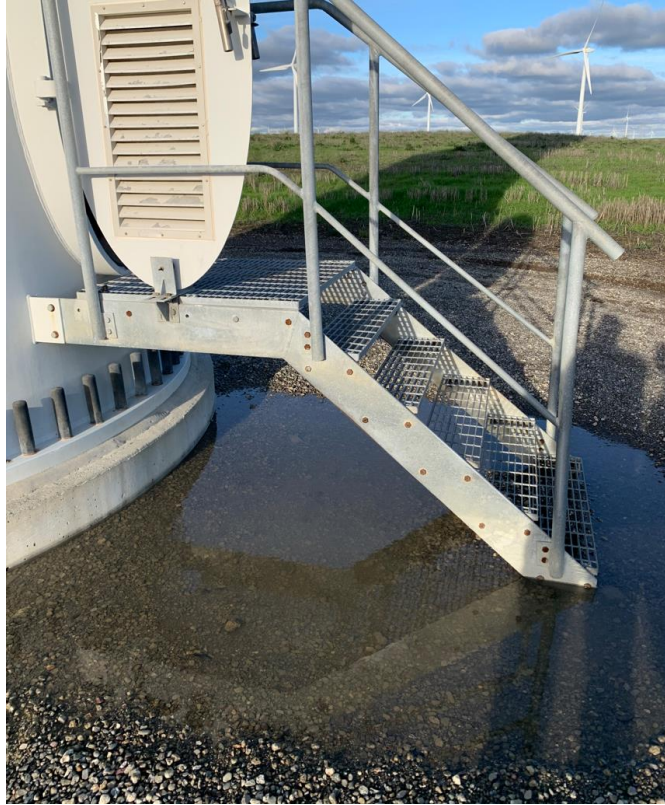
Figure 11. Tower base and stairs of WTG F4.
