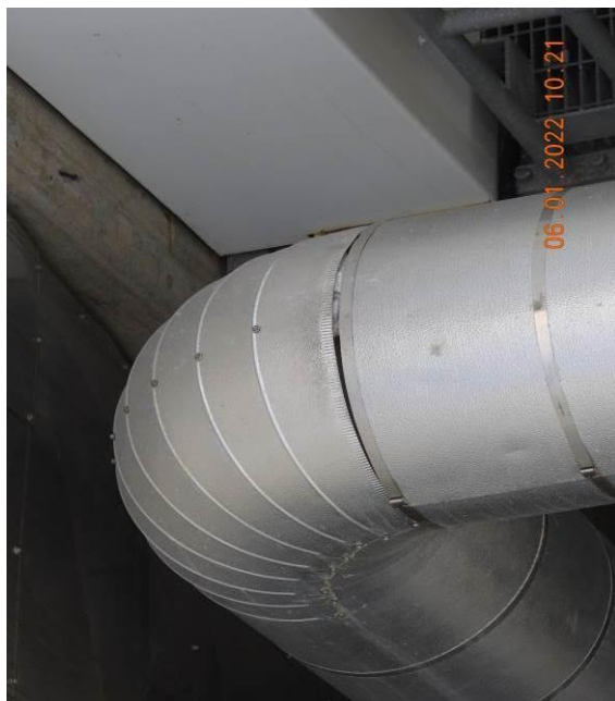
Damaged Insulation
