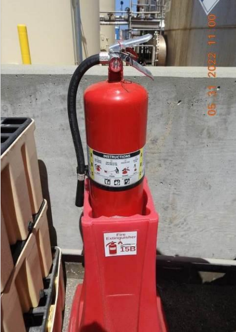
Outdated inspection tag and missing inspection tag
