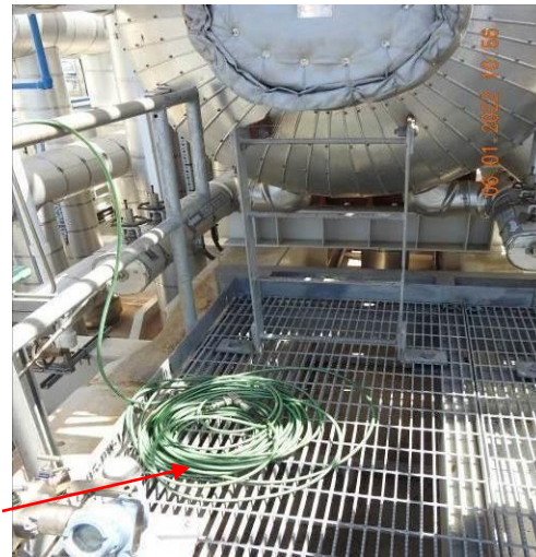
Hoses on the ground
