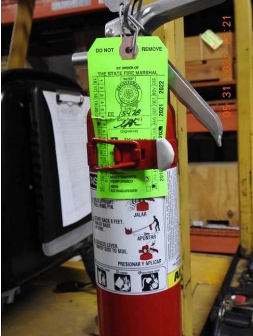
Outdated inspection tag and missing inspection tag
