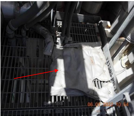
Gloves, pipe joint, insulation cover on the ground
