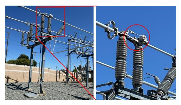
4.3. Exposed ground, broken moulding, transmission pole H29-205 located within the substation.
