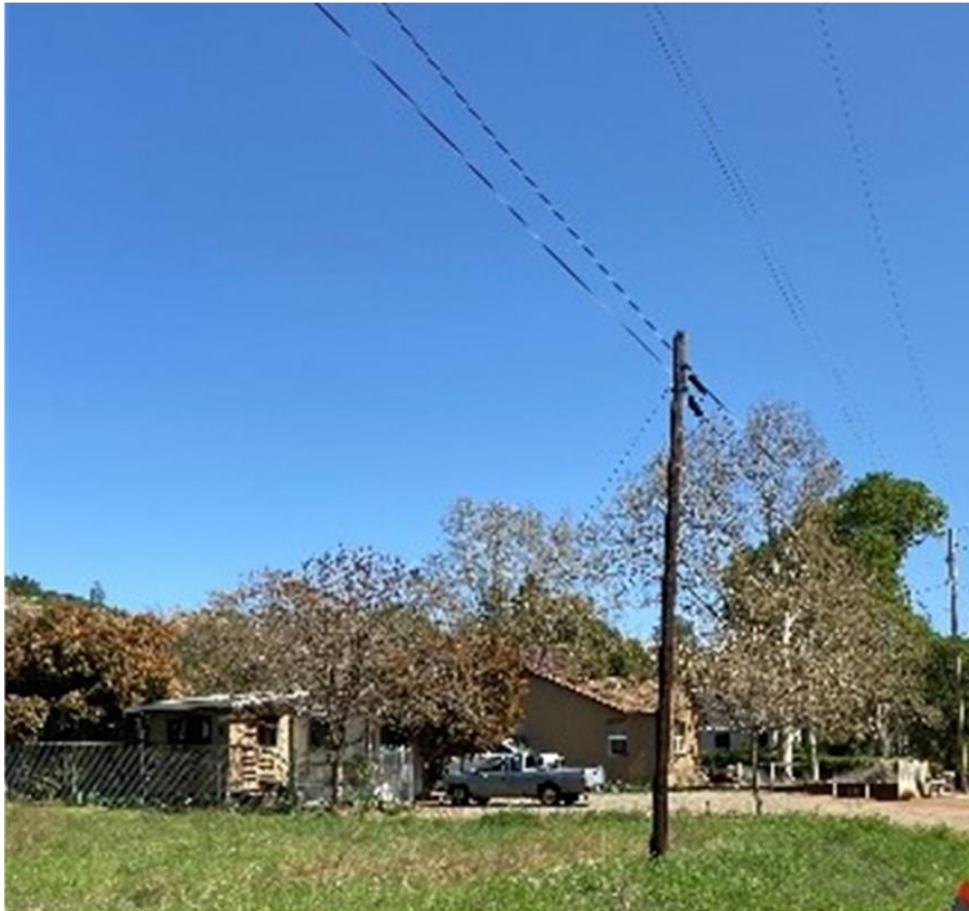
Figure 5: Lack of Intrusive Inspection at Location 5
