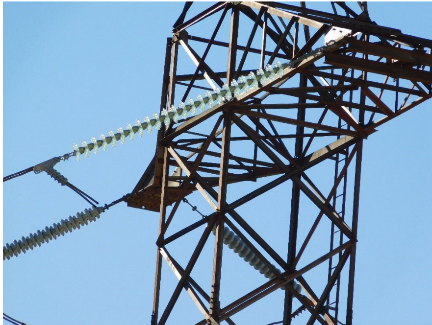
Figure 7: Installation of new insulator strings.
