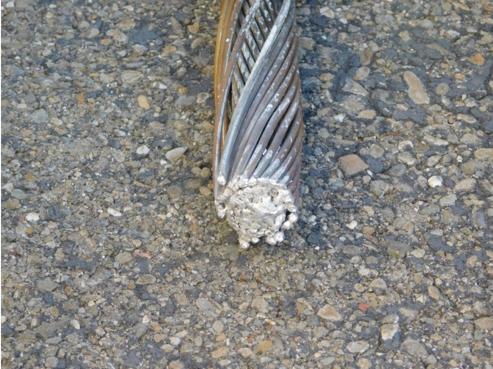
Figure 12: View of the failure point. This is the side of the failure point that was hanging in the air prior to evidence removal.
