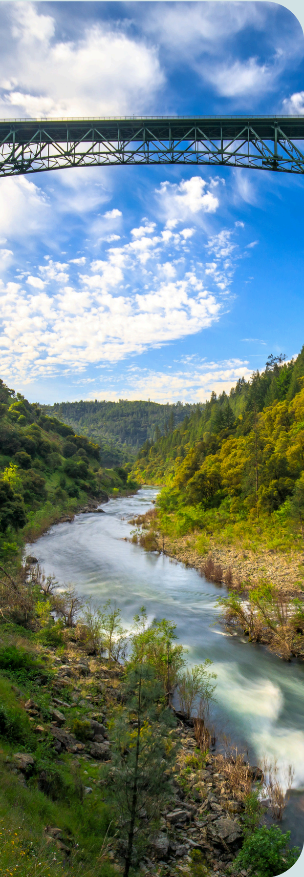
Forresthill Bridge, Auburn
