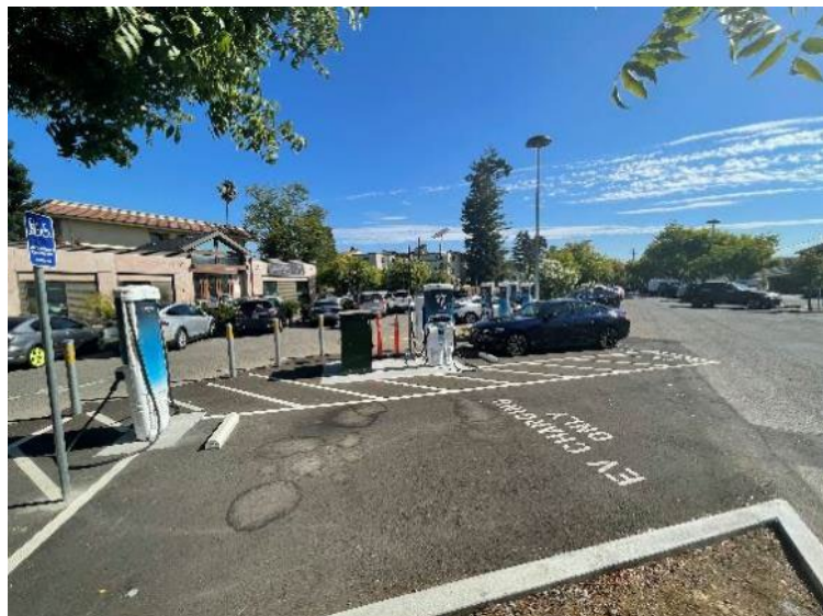
Figure 167. Example of DCFC Charging Layout
